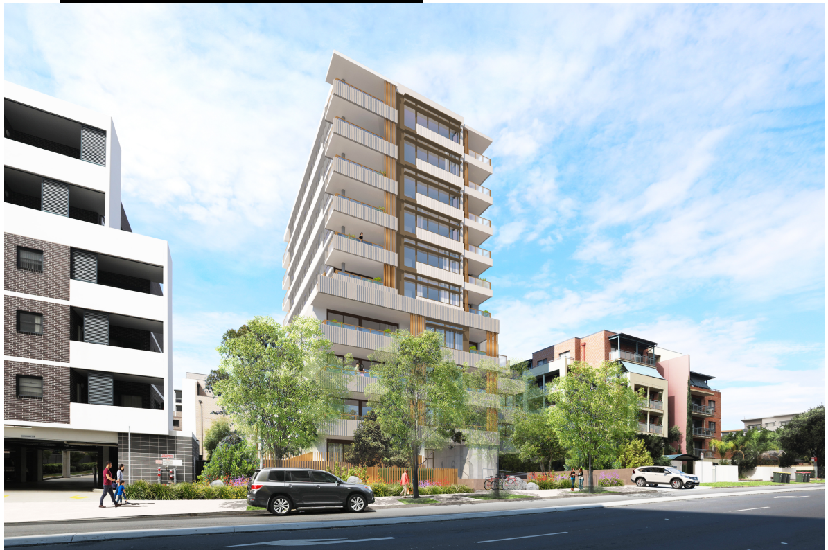
VIEW FROM BIGGE STREET
